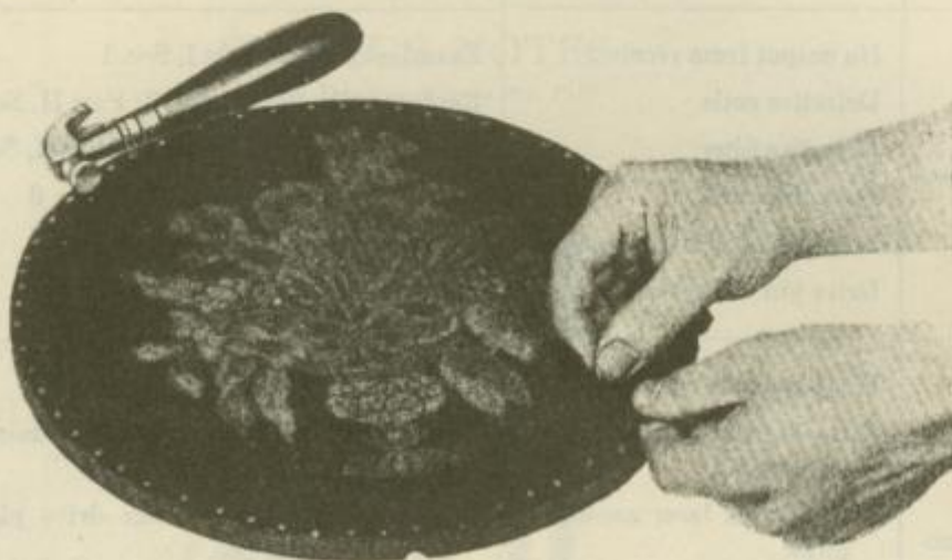
Figure 14—Tacking the grille tapestry in place on the baffle board
