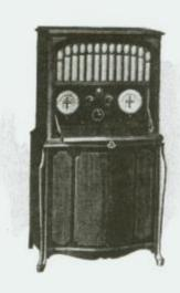
The peer of all Radiolas, Radiola Super VIII, is particularly designed for use in cities and areas local to broadcast stations, where the erection of an antenna is often impracticable, and where an extremely high degree of selectivity is absolutely imperative. The Super-Heterodyne principle, improved beyond any comparison to previously existent designs, provides super-selectivity, enabling one to tune in distant stations under the shadow of a local broadcast station.
